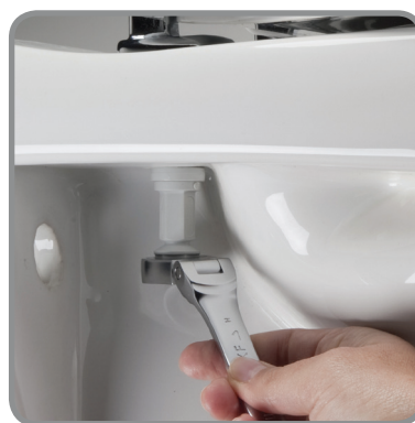
Tighten with Spanner
