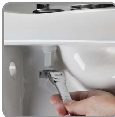
Tighten with Spanner
