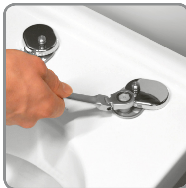
Tighten with Spanner
