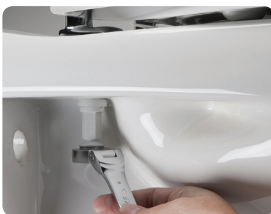
2) Tighten with Spanner
