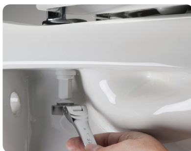
2) Tighten with Spanner
